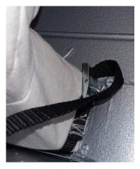
To empty the filter bag the bag needs to be unhooked at the top of the bag holder frame. The ratchet strap should then be loosened.
